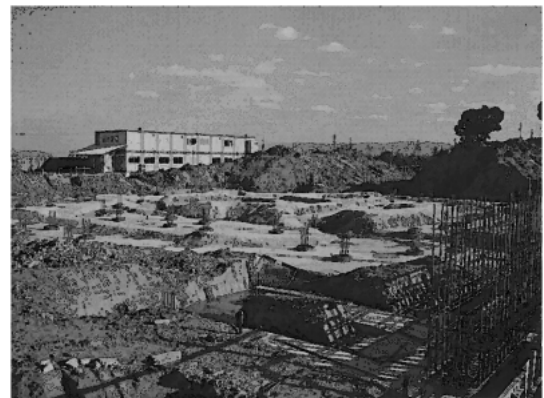
Figure 9. Recent picture of the building under construction.
