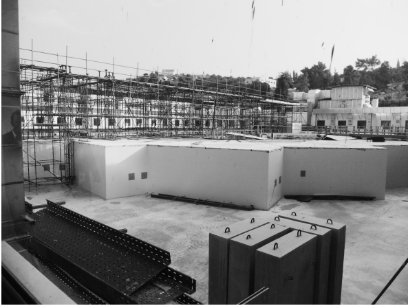
Fig. 3 A photo taken on Dec. 2014 from the second floor of SESAME building. The white structure is shielding for the storage ring but there was no roof and neighboring hill and buildings can be seen.
